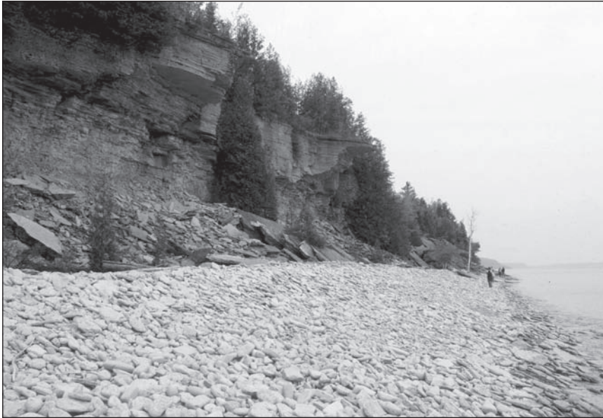
Figure 13.7 Erosion of shale at the cliff toe leading to undercutting and failure of blocks of relatively resistant sandy dolomite, Cape Dundas, Georgian Bay, Ontario. The shale is one of the lower units in the Niagara Escarpment. Note the rectangular jointing pattern in the overlying rocks which controls the size of the failure blocks.
