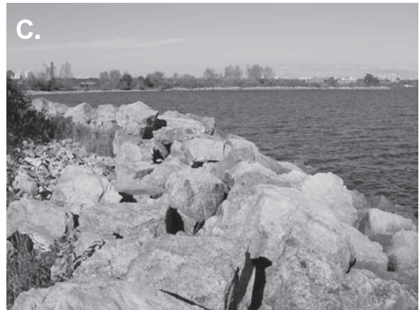
Figure 8.15 (A) Evolution of a log spiral beach down-drift from a seawall on the Illinois shoreline of Lake Michigan (after Terpstra and Chrzatowski, 1992); (B) artificial headlands and crenulate bays on a complex landfill feature, Toronto waterfront, Ontario, Canada; (C) ground view of the armourstone structures forming one of the headland structures in (B) with the Toronto skyline in the background.
